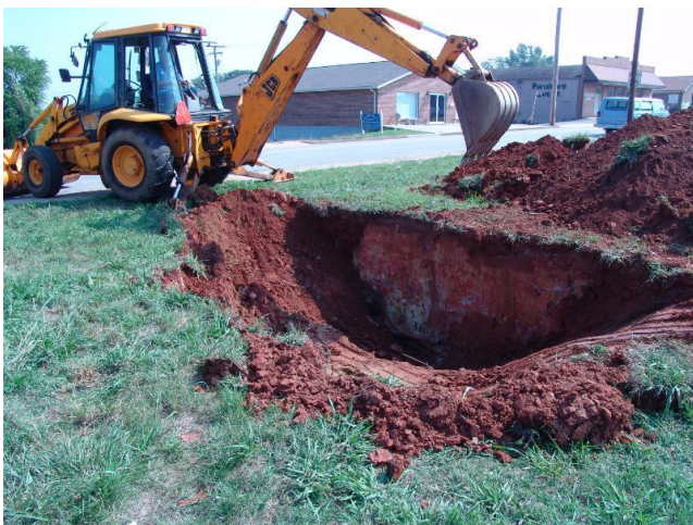
Baldwin Building foundation, exposed using heavy equipment. The highly compacted soils of this urban setting made hand excavation nearly impossible.
