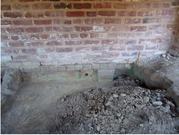
This photograph of the Selden addition foundation shows that the bottom course of header bricks rests directly on (almost) sterile subsoil.
