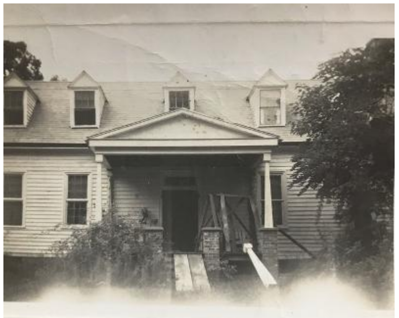
Ca. 1947 repairs in progress on the south porch at the front of the Manor House. Note the much taller brick piers and brick steps that are no longer there.
