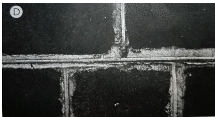
Figure 7. Mortar fragment with a tuck point finish (left) excavated from Feature 40 (Germanna Archaeology), and (right) tuck point joint example shown in The Chesapeake House (Carson 2013).
