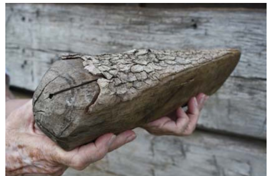
Closeup of a pine log wedge used as a supplemental means of chinking for the log structure.
