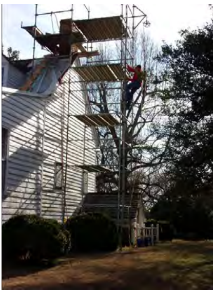
Scaffolding around west chimney. Photo by Martha Williams.
