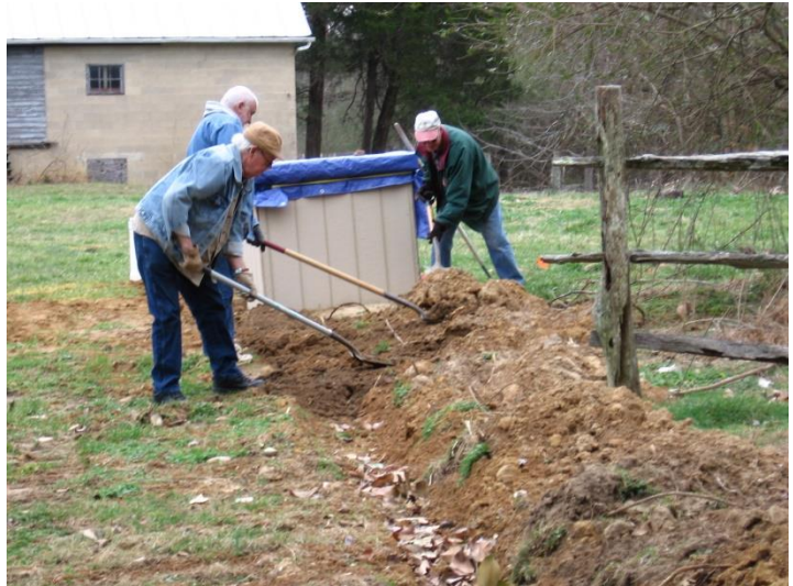
Backfilling the water line trench at Kittiewan.
