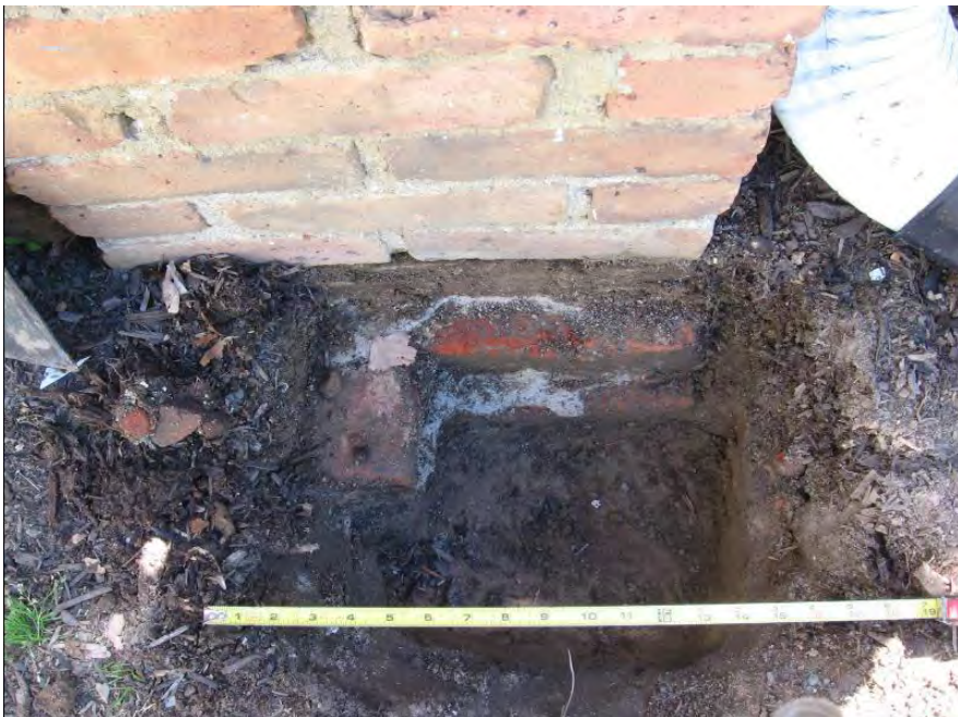
Excavating an underground drainage channel revealed an earlier brick pier support for the front porch.
