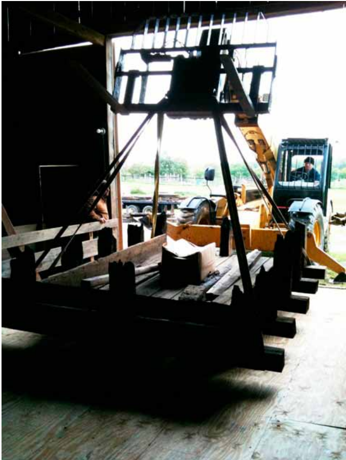
Carefully positioning mill components in Clermont's barn.
