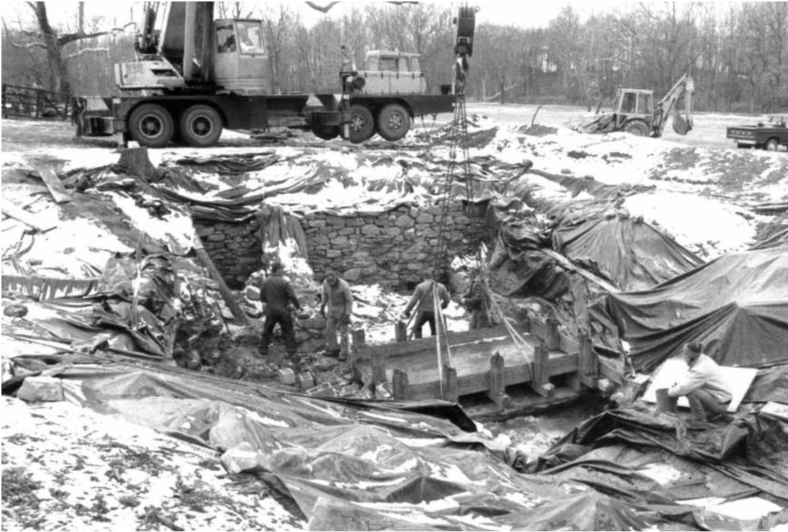
Removal of forebay from stone foundation of Woolf's Mill.
